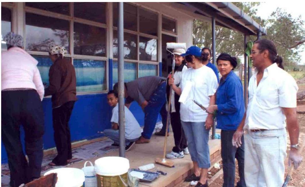
Parent Workgroup in action - painting the foundation phase blocks
