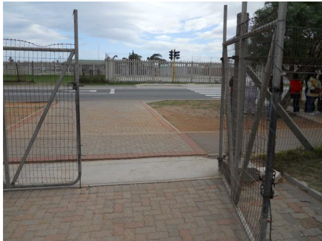
Easy target for unauthorized entry – the previous school gate was old and had no secure locks
